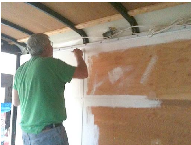
Chuck begins the base coat of paint. The white color will brighten up the inside by reflecting existing light better.
