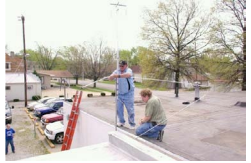
Kevin and Steve put the ground plane on the Gap Titan.
