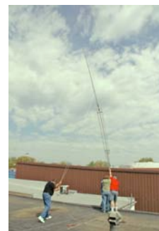
The rest of the crew heads up to the roof to mount GAP Titan DX and a home-brew 160m off-center fed dipole.
