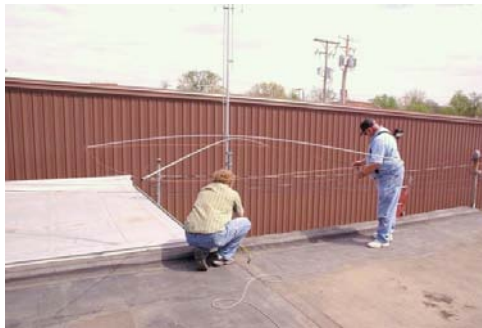
Kevin and Steve put the ground plane on the Gap Titan.
