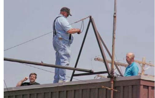
The air conditioner behind Melody and the tripod that Steve's working on are the endpoints for the 160 meter dipole.
