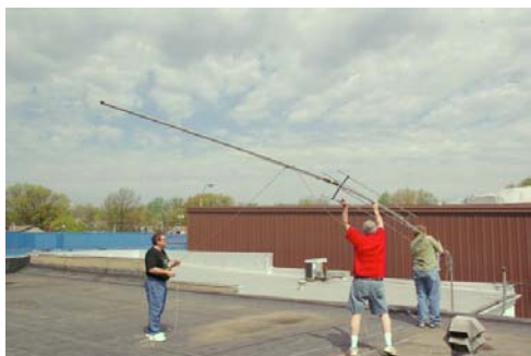
The rest of the crew heads up to the roof to mount GAP Titan DX and a home-brew 160m off-center fed dipole.
