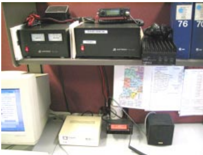
This is how we, here at Illiana Skywarn, thanks to the new 440 linking system, get our audio information - Amateur Radio Station W9NWS, located here inside the National Weather Service office.
