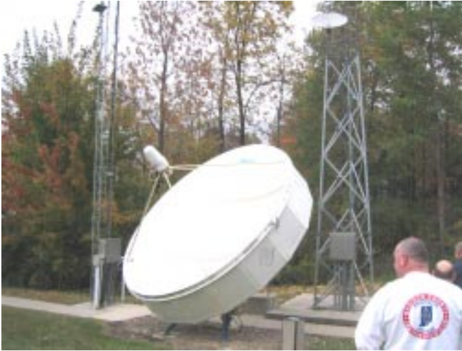
This is how we get the visual information from the NWS. This is the data uplink to satellite.
